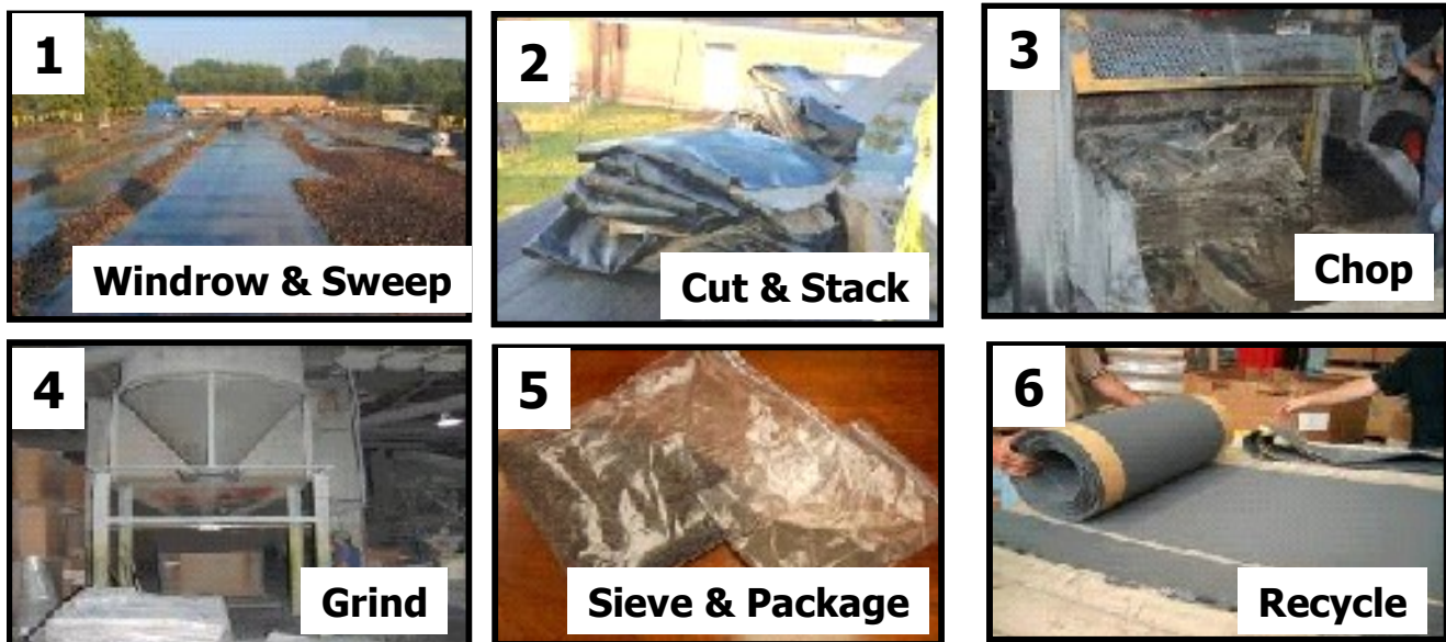
Figure 4: Ballasted Roof Recycling Steps
