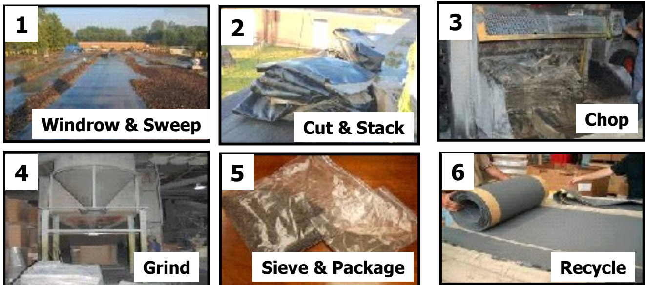
Figure 4: Ballasted Roof Recycling Steps
